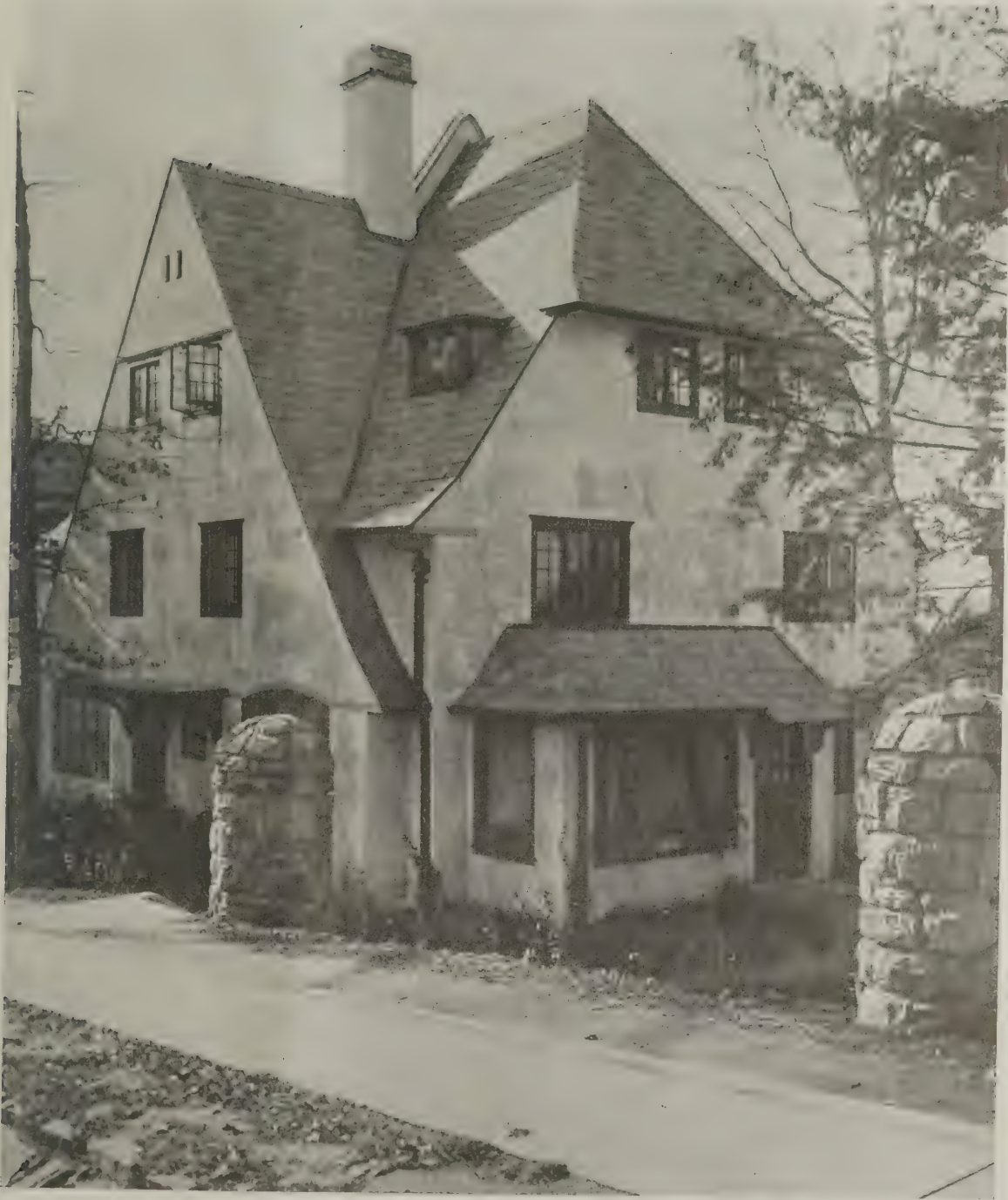
SEMI-DETACHED TWO-FAMILY HOUSE AT SOUTHERLY END, OAK COURT TERRACE, BRONXVILLE, N. Y. BATES & HOW, ARCHITECTS. NOTE FIRE WALL DIVIDING THE TWO SECTIONS, WHICH EXTENDS ABOVE ROOF IN BACK OF CHIMNEY
